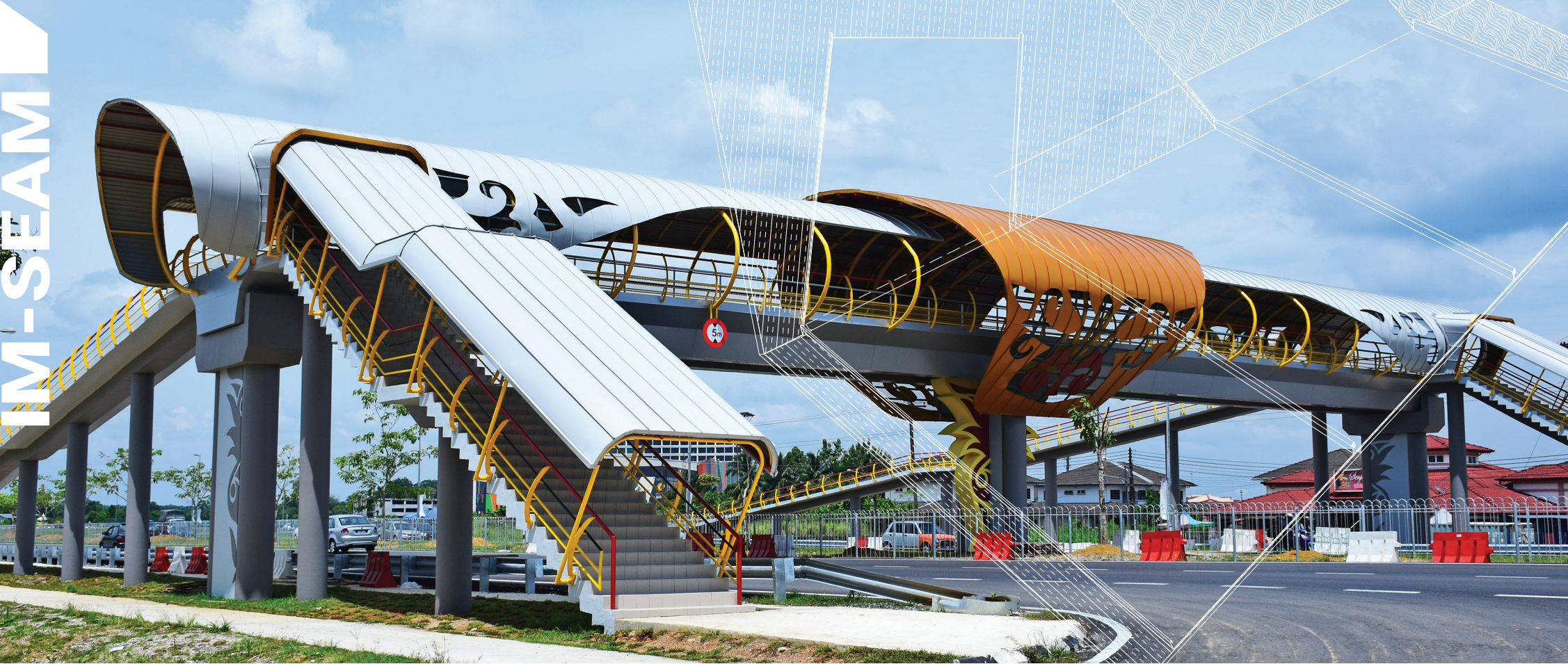
■ Samarahan Pedestrian Bridge, Samarahan (2016)
