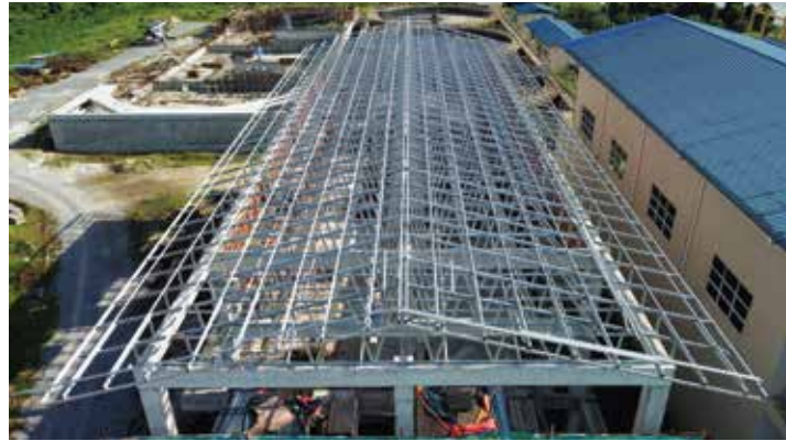
■ Kuching Centralised Sewage Treatment Plant, Kuching (2022)
