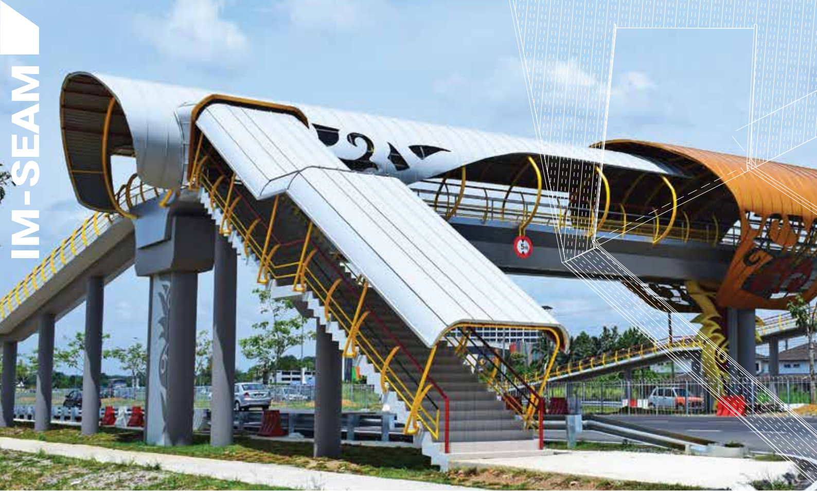
■ Samarahan Pedestrian Bridge, Samarahan (2016)
